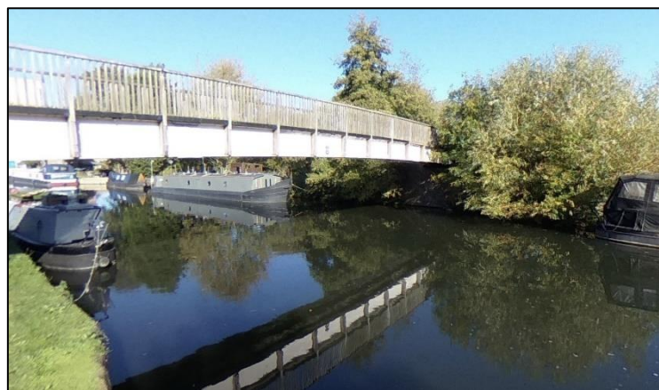
One of the bridges leading to Tumbling Bay
