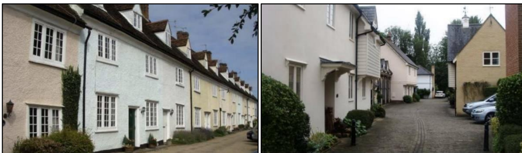
Images show: 17 th century nurses' cottages for Bluecoat School and Christopher Court picks up on built elements (materials, colours, architecture) from the surrounding context
